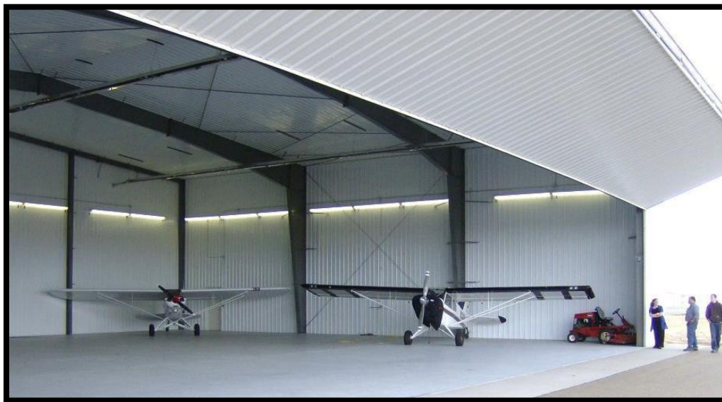
Figure 10.6: Hangar at Baker Municipal Airport
